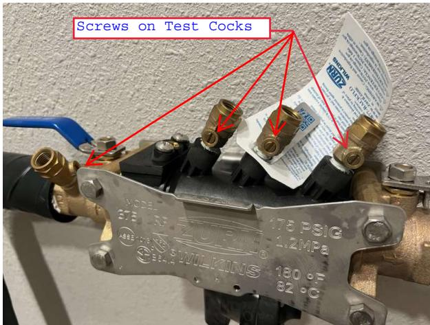
5. Once water subsides, turn the screws on each test cock so they are at a 45-degree angle to the direction of the Test cock.
