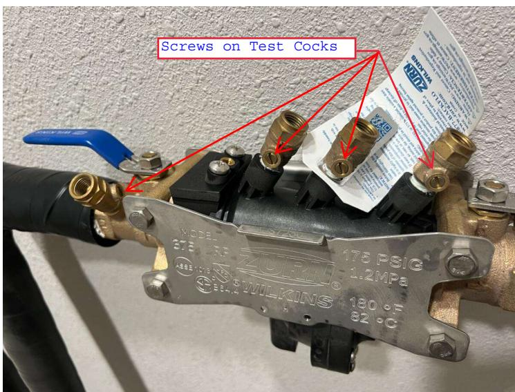
6. Turn Handles on the backflow device to a 45 degree angle and place plastic caps back on each test-cock.
