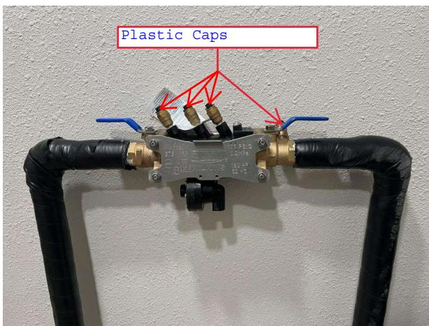
4. Open the bleeder valves (Test Cocks) to a horizontal position:
