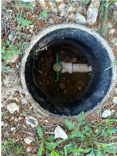
**3. Remove (unscrew) the plastic caps from the Test Cock**
