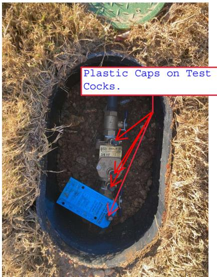
**4. Open the bleeder valves (Test Cocks) to a horizontal position:**
